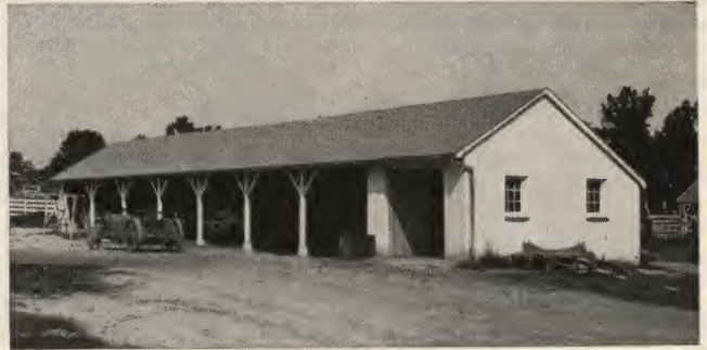
An attractive and serviceable implement shed with enclosed repair shop on one end.
